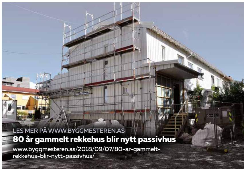
Endeleiligheten i Lørenfare under rehabilitering sommeren 2018.
