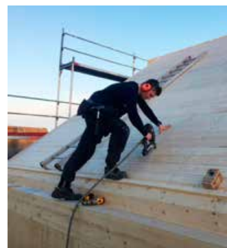
Jone Soldal spikrer takelementer.
